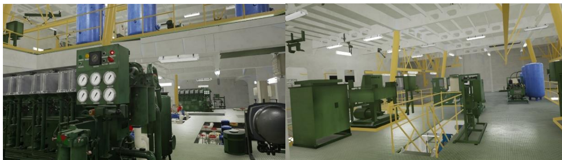
Figure 4. Ship engine room in the VR environment
